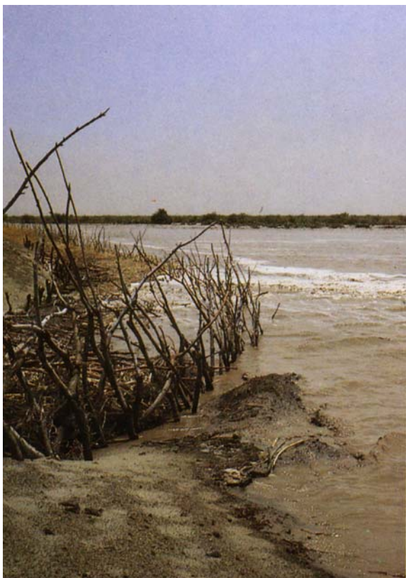
Local embankment protection
