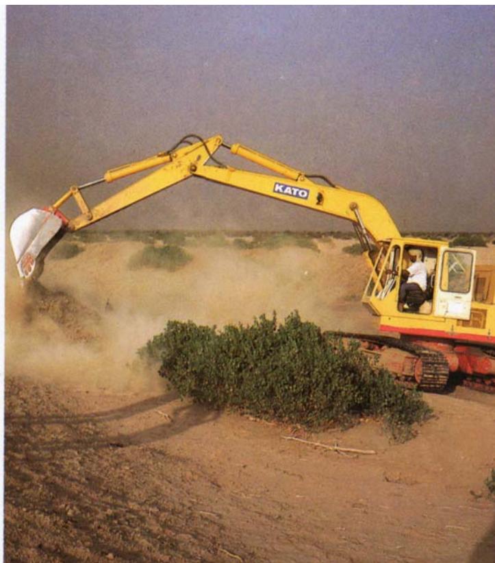
Reconditioning of smaller canals
