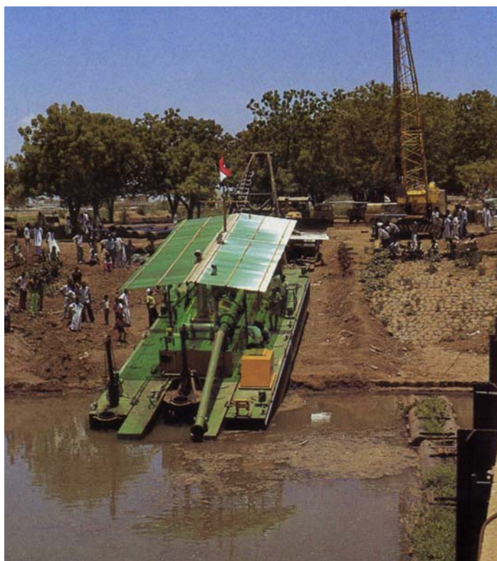
Launching of the Cutter Suction Dredge
