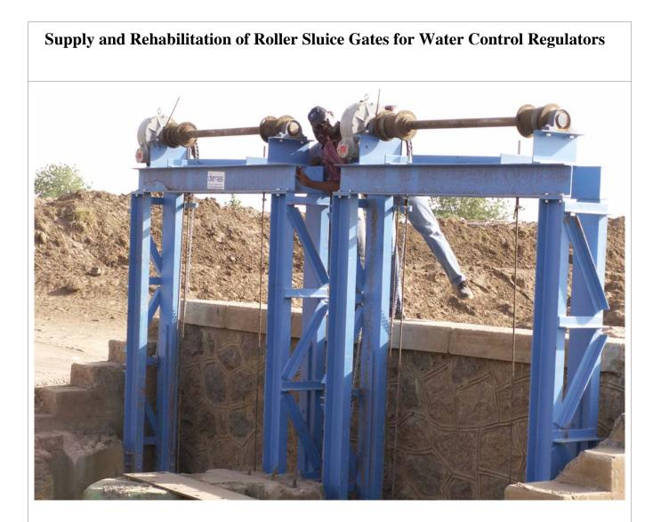
DEMAS did win an international tender by the Ministry of Irrigation and Water Resources in the Sudan for the supply and rehabilitation of Roller Sluice Gates (RSGs) for water control regulators in the Gezira Irrigation Scheme. The project includes design and supply of 26 existing RSGs. Furthermore, missing parts need to be supplied for another 23 RSGs, which were supplied some time ago and stored at the client's yard in Wad Medani.
