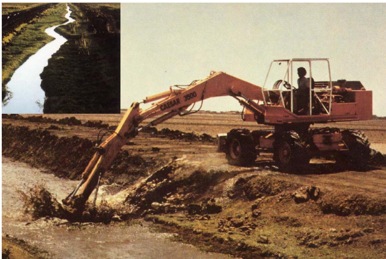
Inset: canal before rehabilitation
