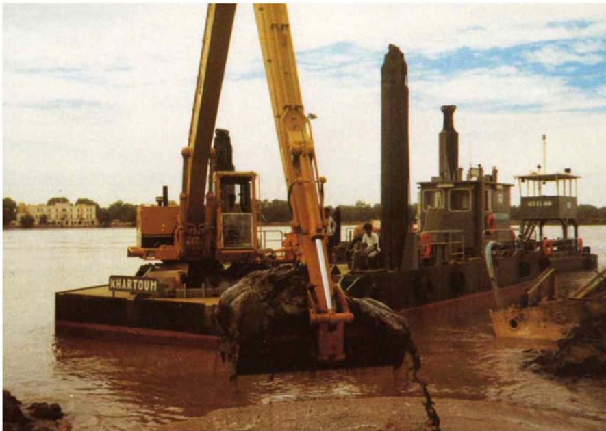
backhoe dredge 'Khartoum' during trial run
