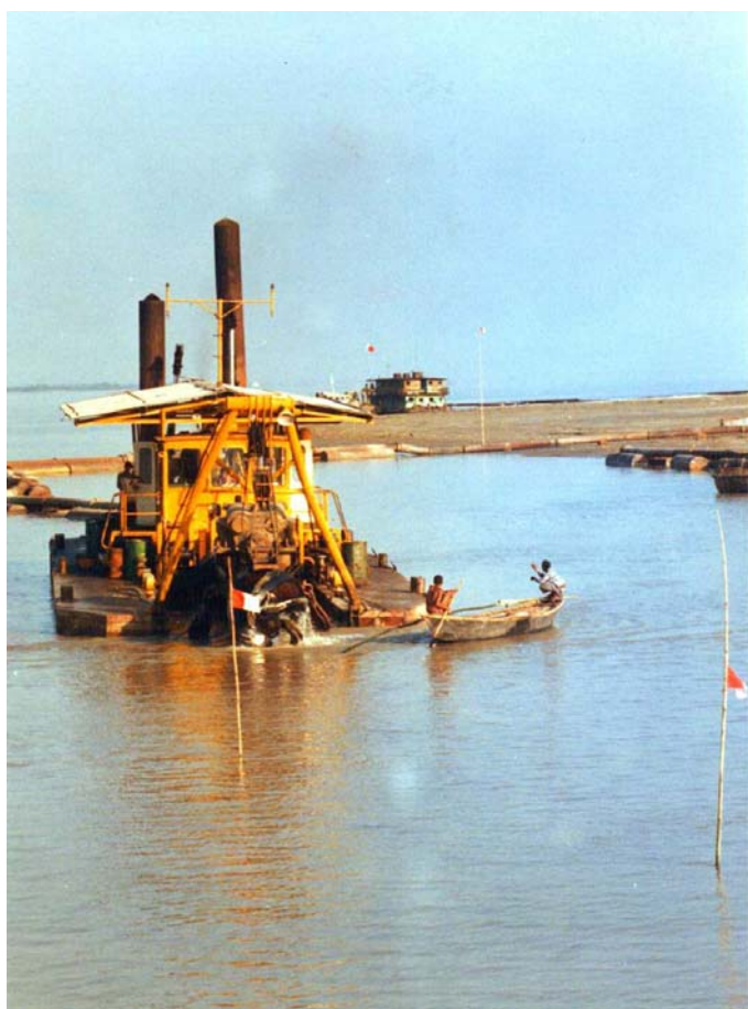
Dredging in Barisal Port
